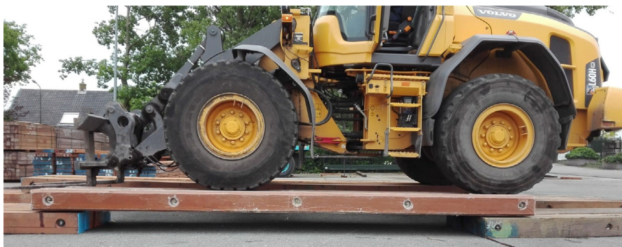
FIGURE 8 Crane mat made of EoL composite tested in practise.
